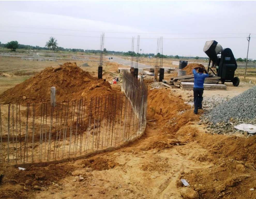
Left side of Front compound wall- Final lift reinforcement works under progress
